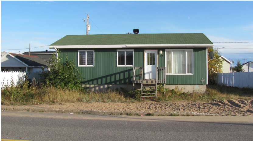
Figure 9: bungalow typique de Uashat
