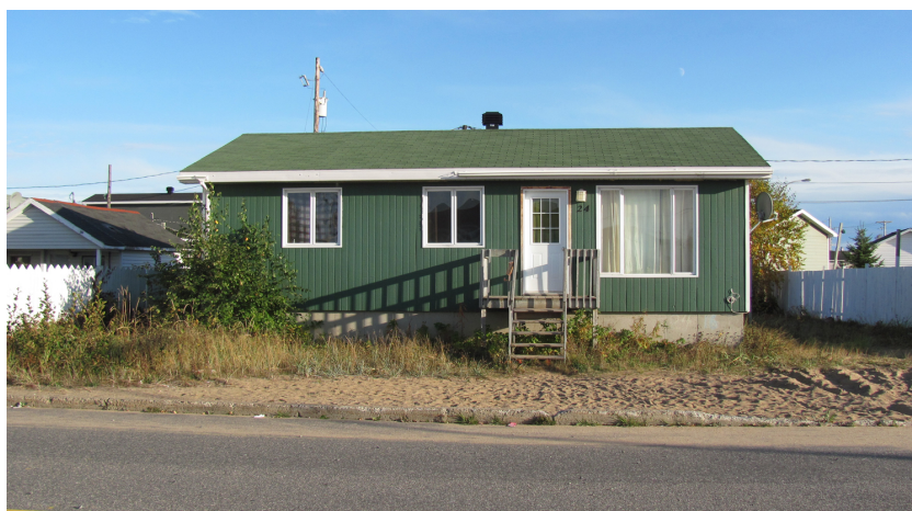
Figure 9: bungalow typique de Uashat
